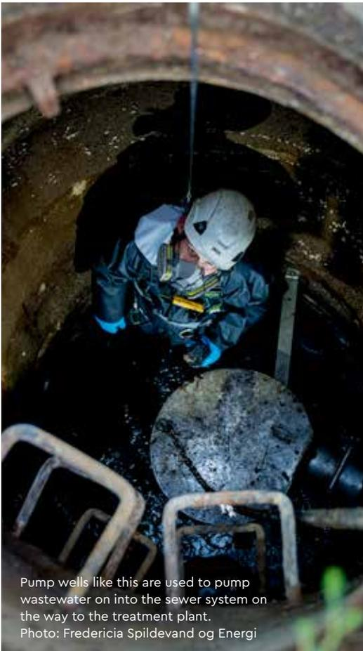
Pump wells like this are used to pump wastewater on into the sewer system on the way to the treatment plant.
